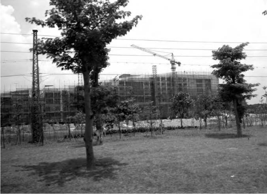
Plate 6.4 Songshan Lake industrial park under construction (source: Lin (2006), p. 49, Figure 8).
