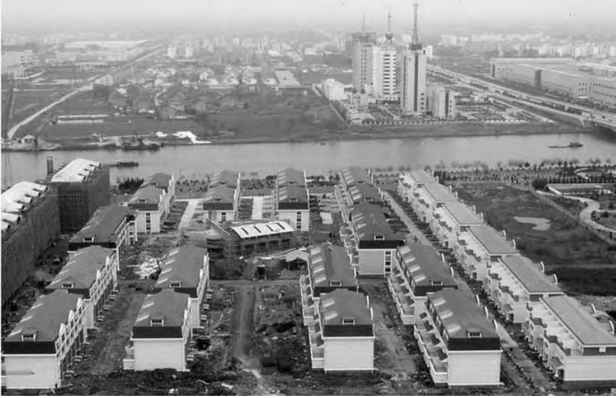
Plate 8.5 New high-tech factories and other buildings in the kaifaqu , Kunshan.
